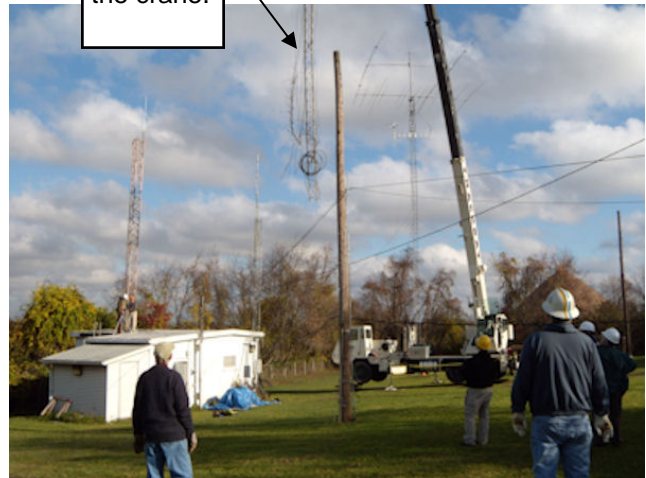
5. The tower free and moved by the crane.
