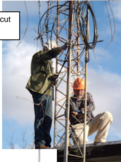
2. Next, the crane sling had to be connected to the top of the tower, but, not on the 2m antenna.
