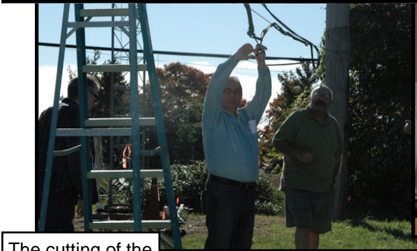
The cutting of the guy wires to drop the damaged tower Oct 2009
